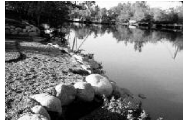
A steep river bank was regraded and stabilized with habitat enhancing boulders at Clark Park on Chicago's north side.
