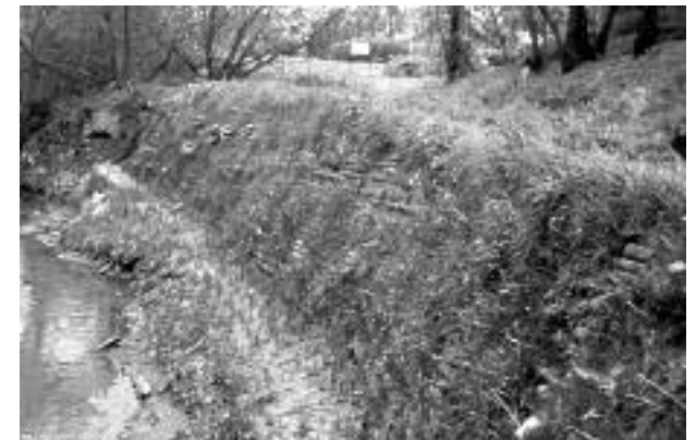
A steep eroded wall was rebuilt with plants and a "live crib wall" on Johnson Creek, Portland, Oregon.
