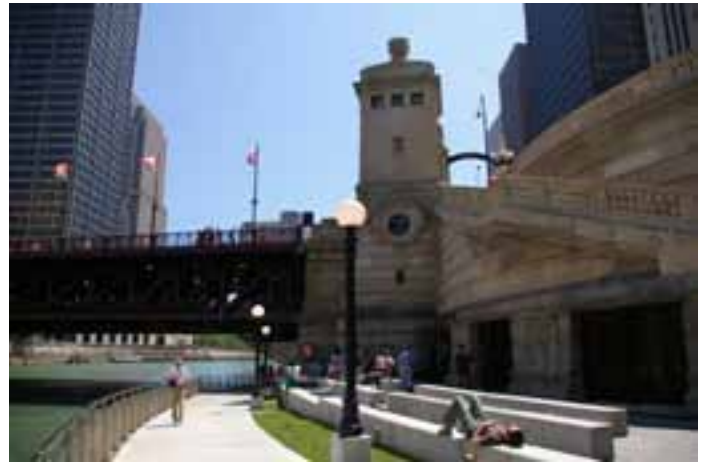
Friends' Bridgehouse Museum now anchors the new Chicago Riverwalk downtown.
